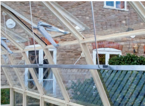
The main structure is now complete: the glass is slipped into place and shelves are fitted
